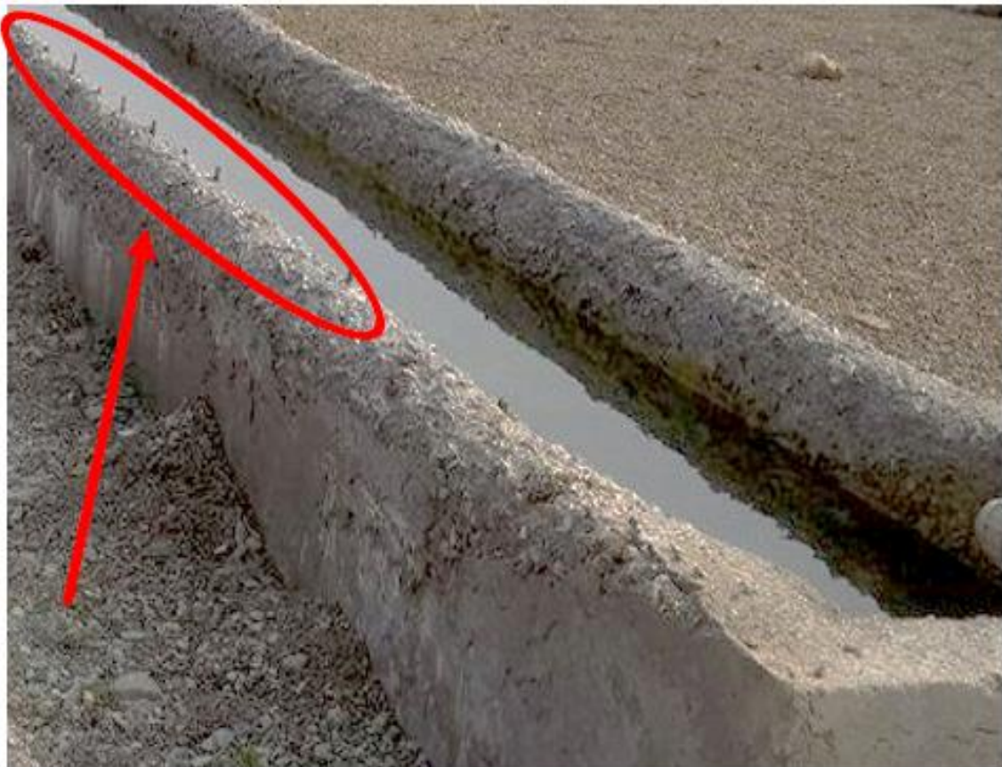
Water Point at Marneuli BSP
