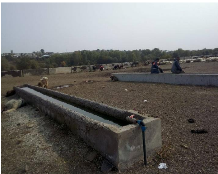
Water Point on Marneuli BSP
