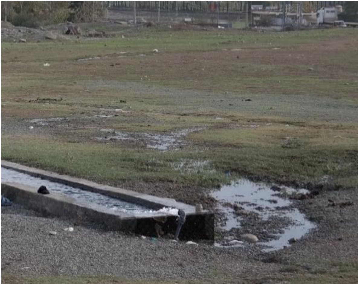
Water Point at Rustavi BSP
