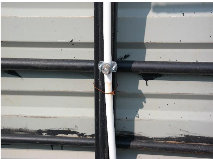
Cattle Shower nozzles at Signagi BSP
